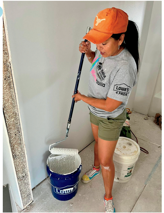
HFHCC HOMEOWNER IRMA WORKING ON HER HOUSE
